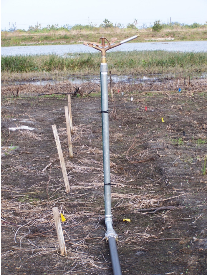
Figure 4.1 and 4.2. Irrigation system on one of the tree islands showing t-valve (top) that diverts water to each of the 2 standpipes and nozzles on each tree island (bottom) as required to partially satisfy Task 2a.
